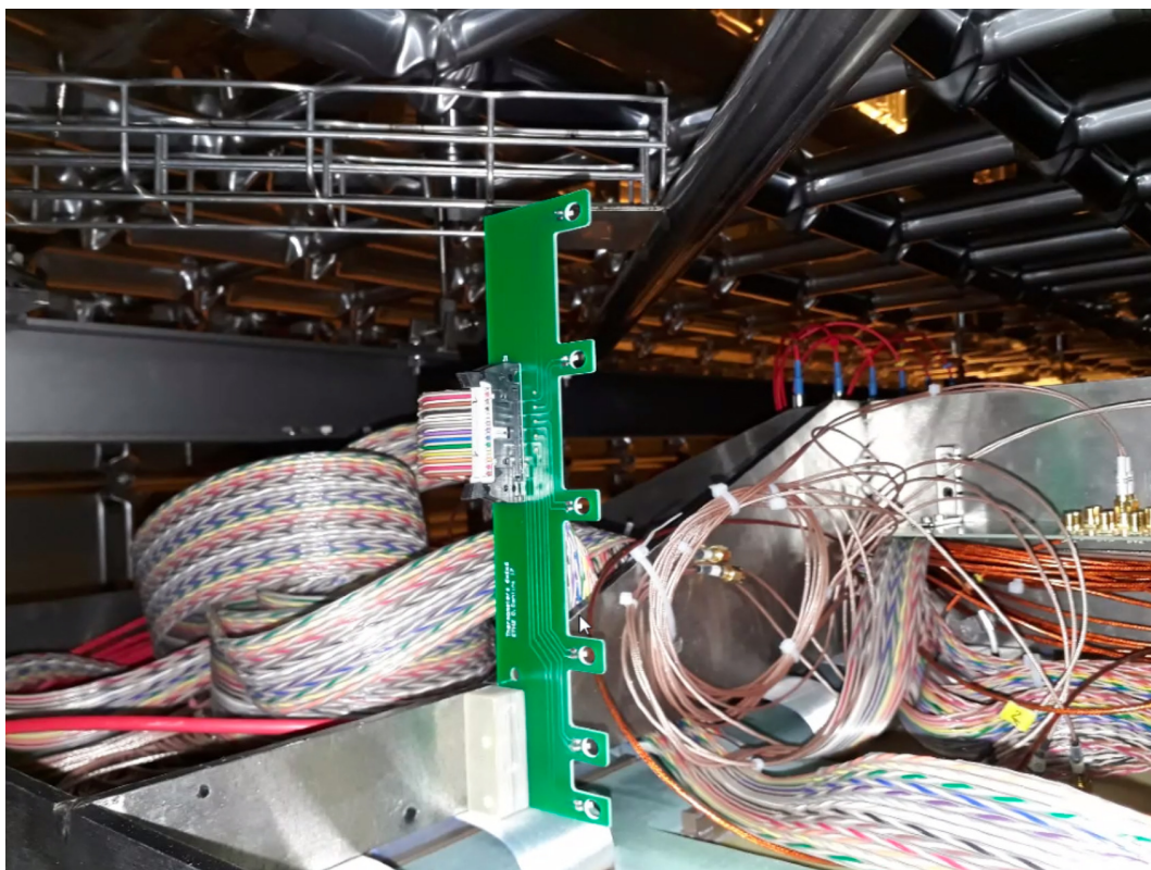
Figure 1.13: Vertical array of temperature sensors in ProtoDUNE-DP.
