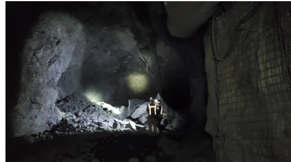
Excavation to full section in North Cavern
