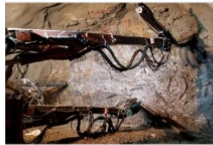
1. Drill Blast Holes
