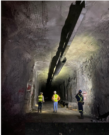
Installing and protecting South Cavern monorail
