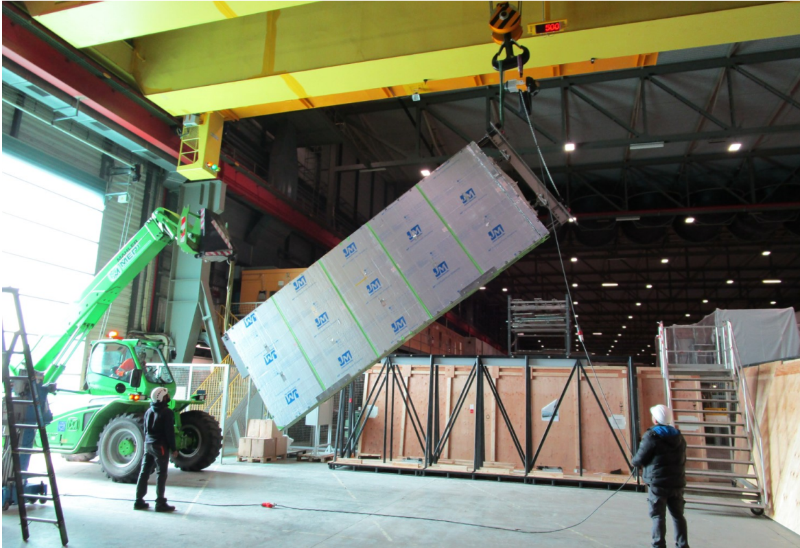
Figure 6 - A ProtoDUNE-SP APA being rigged from horizontal to vertical using a similar technique at CERN.
