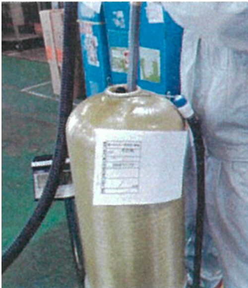
Remove existing resins
