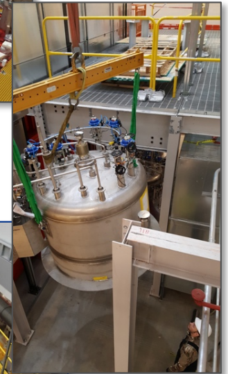
Rigging valve boxes
