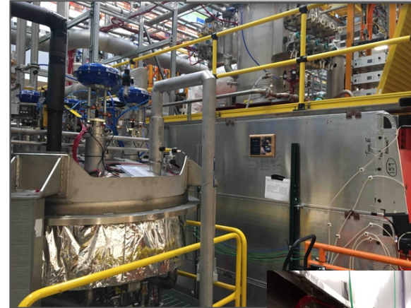
CRT North wall
