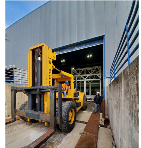
Atf being pulled out of DAB.
