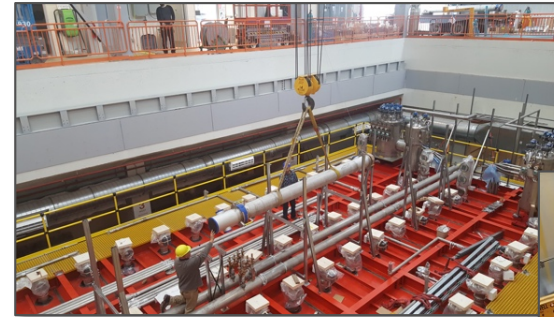
Rigging valve boxes
