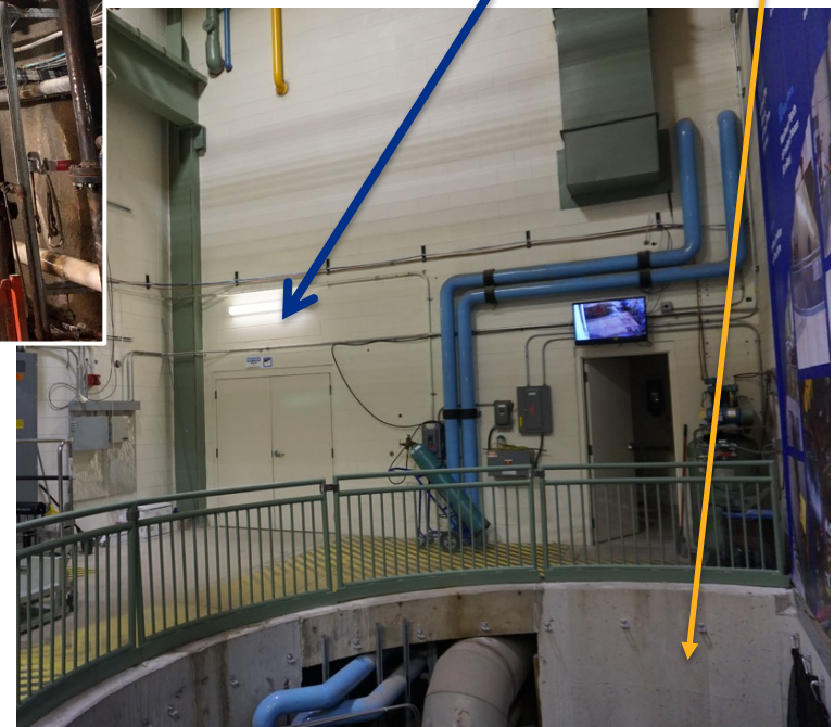
Laser lab being built behind this wall.
