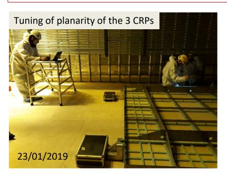
The planarity of the CRP is measured and adjusted on 50 points and 2-3 iterations.
