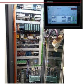
The system can act for 1 to 4 CRPs together as a master system. All the motors will get the same position change Feedback loop is provided by the level meter information.
