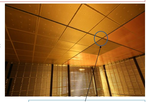
The procedure failed in improving the horizontality because of the absence of information from 1 corner
