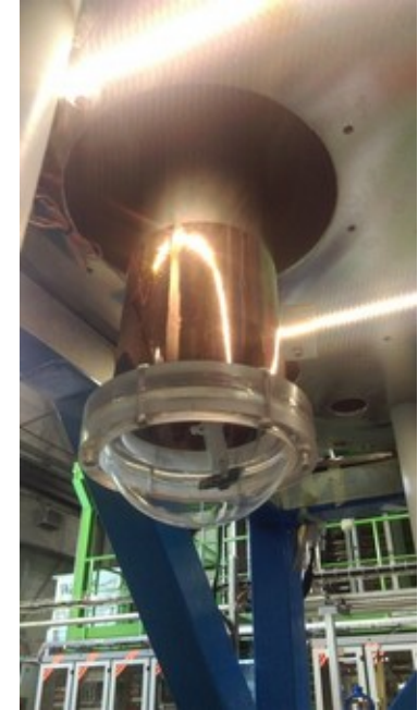
Photo of steel tube intrusion at bldg 182.
