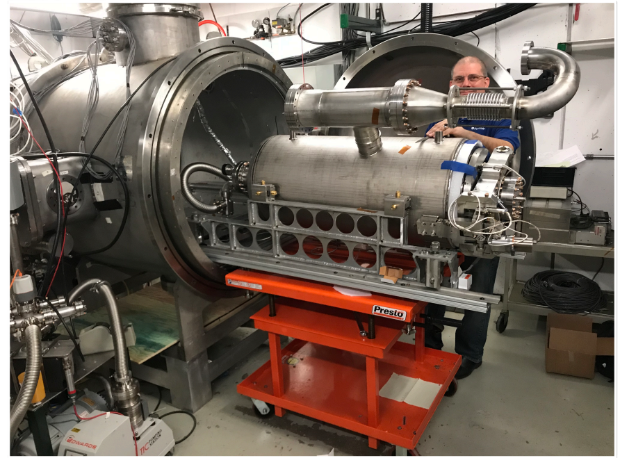
Installation into STC, B9A-AES-010
