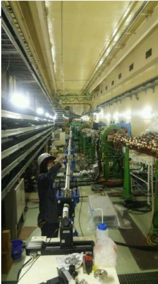
X-ray beam line under construction at LER
