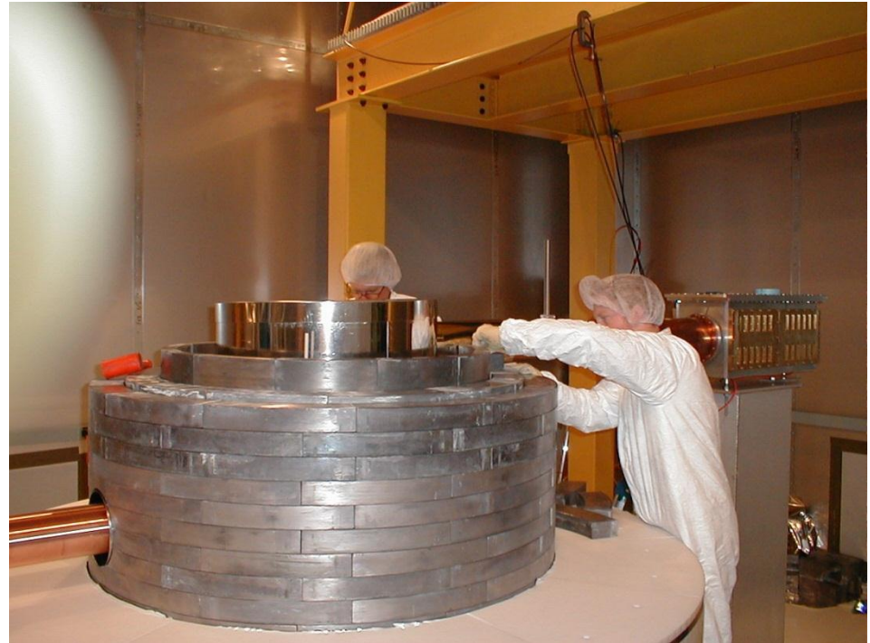
SuperCDMS Shielding installation
