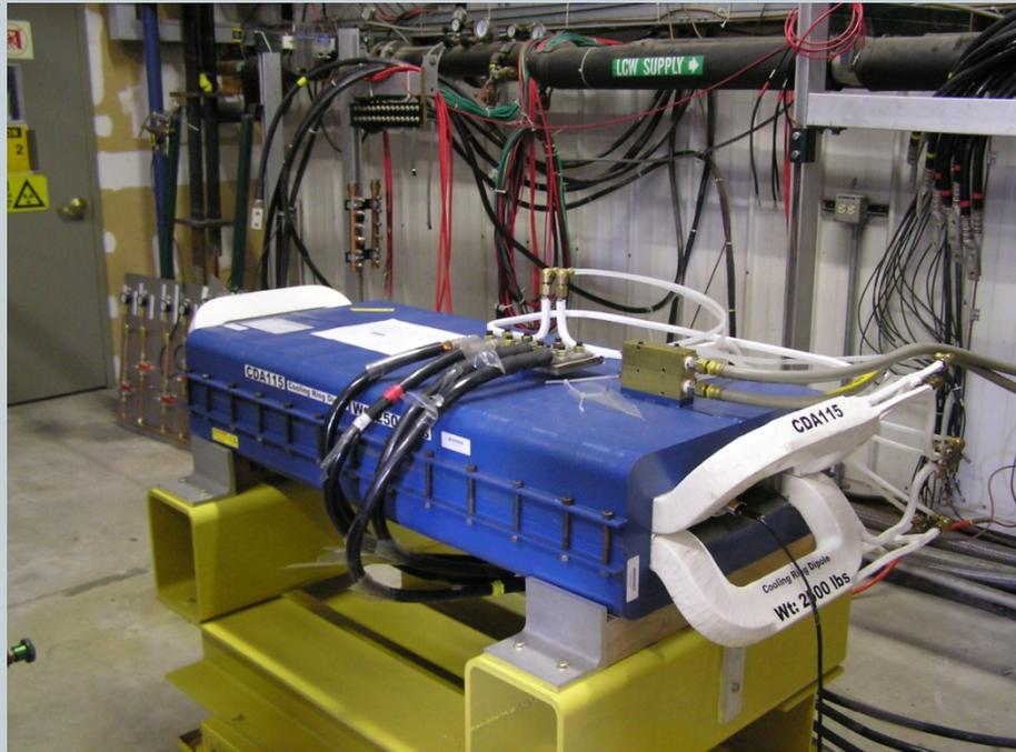
Power Supply that will be used to ramp the magnet. The supply is 75v@1000a.
