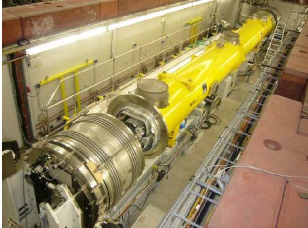
CMTS Outer Bellows pulled back to access piping
