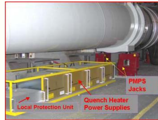
Quench Heater Power Supply (QHPS) HDS units 5500
