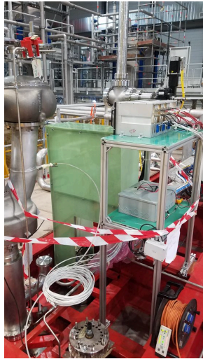
PrM Rack for PrM Front-End electronics and Light source on cryostat
