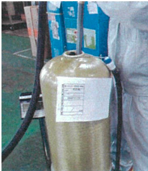
Remove existing resins
