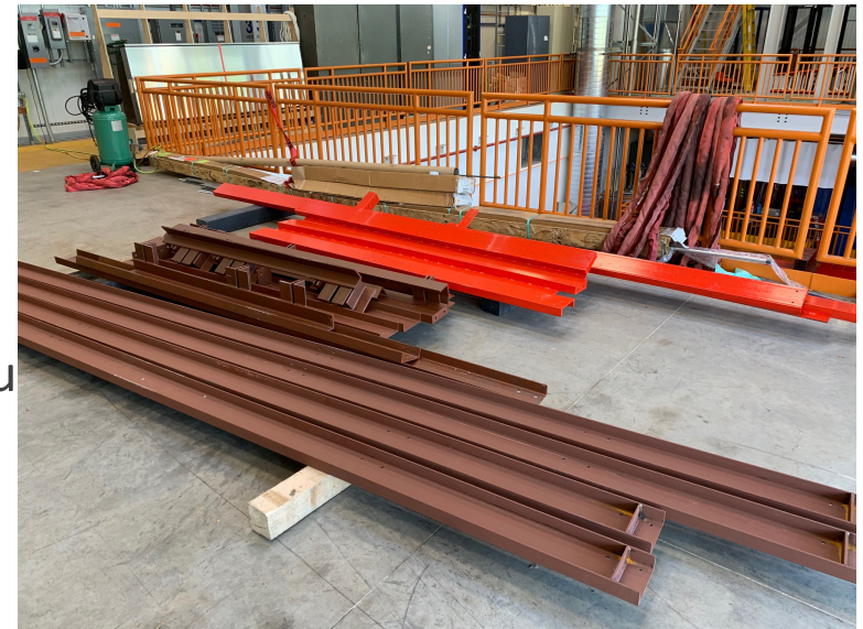
Stair and decking structure ready to install
