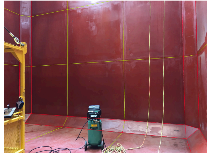
Weld leak checking
