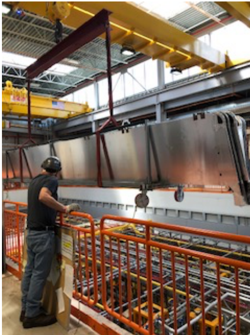
Transporting the modules
