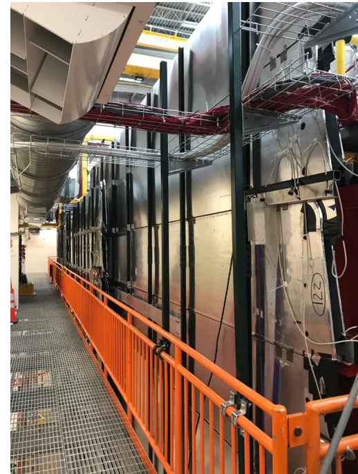
East walls complete
