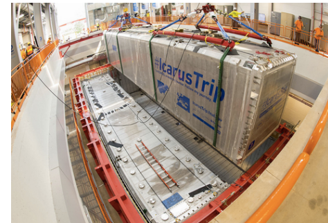
Figure 2: Installation of the two modules of ICARUS.
