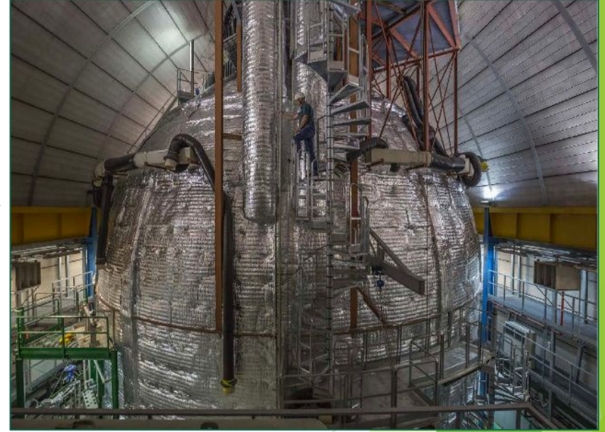
After the thermal insulation (Early 2016)
