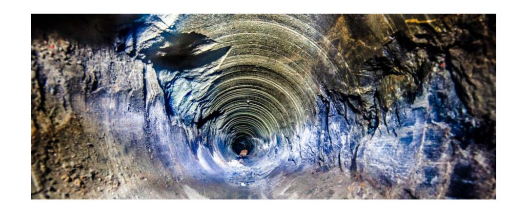
View along the long axis of a horizontal borehole with breakouts showing effects of stress – 4850 Level SURF
