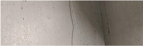
Piped cleared away, penetration capped and filled with sand (+ 3' poly beads)
