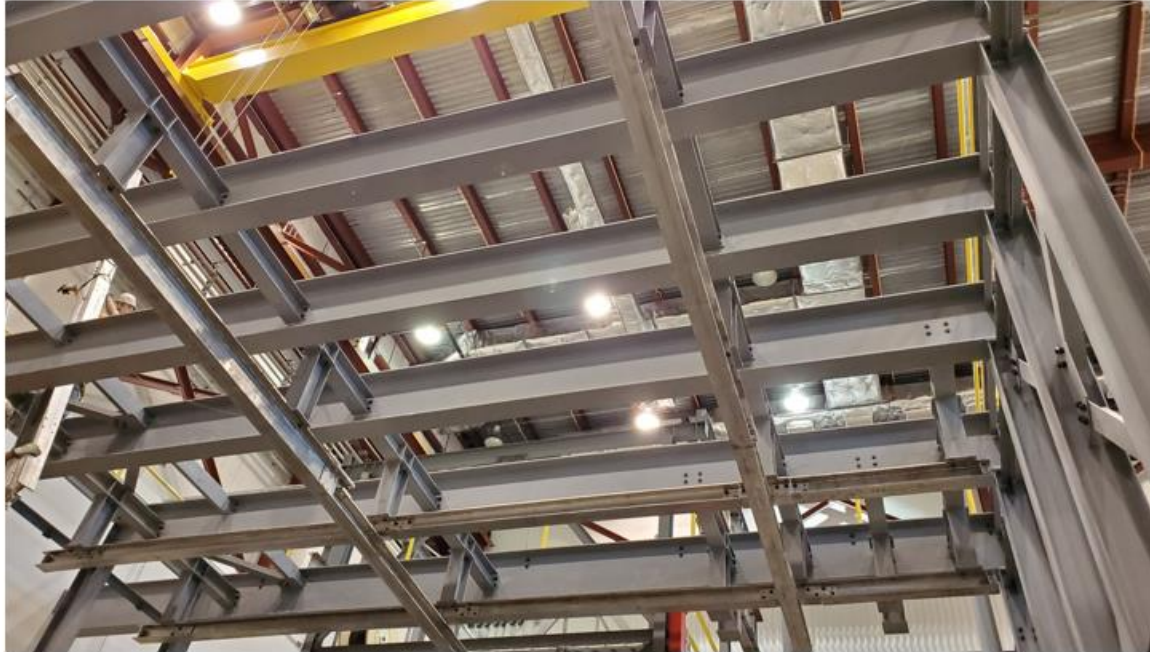
Ash River Phase 2 DSS Load Test Plan William Miller Tom Wieber University of Minnesota
