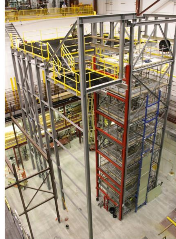
Phase 2 DSS support structure at Ash River
