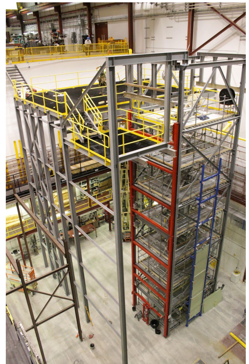
Phase 2 DSS support structure at Ash River
