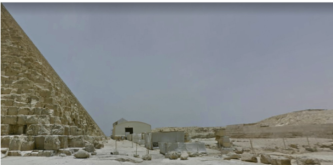
Figure 7: Ground-side view of the south side of the pyramid (looking east), near the face.
