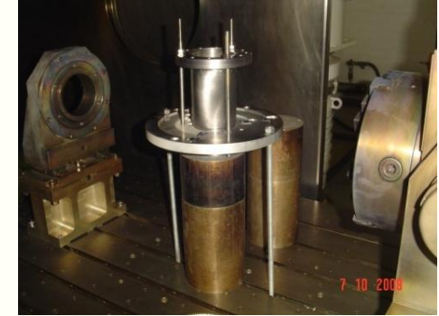
Pipe Flange welding
