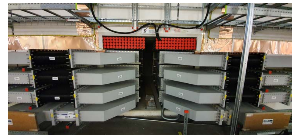
SCL RFDS, Tunnel
