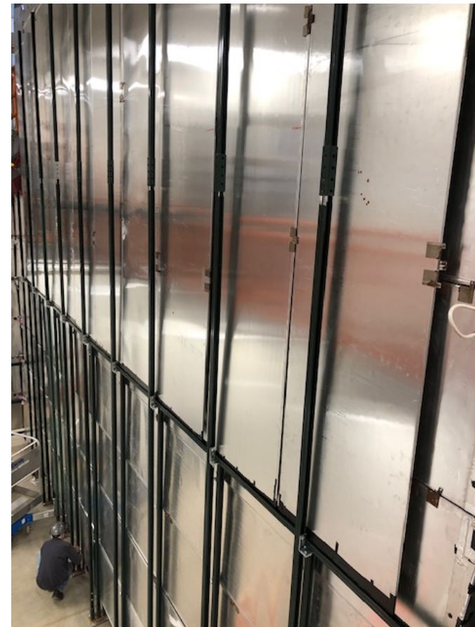
CRT South wall complete
