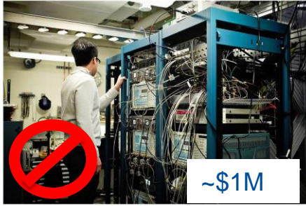
No Missed Connections Jerry M. Chow, PhD, manager of theory of quantum computing and information at IBM Research, inspects the cables connecting a vast array of microwave equipment powering quantum computing processors in the lab.
