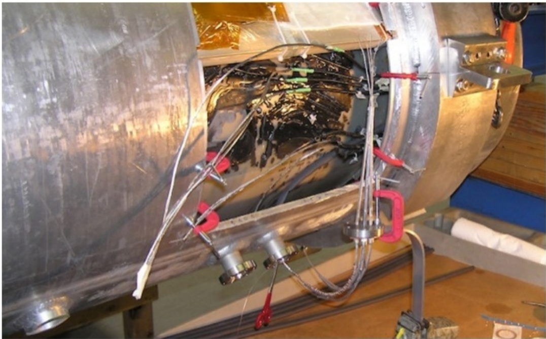
Figure 6: Repair and stabilization of the Magnet 2B cold leads.
