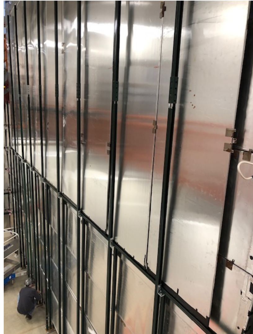
CRT South wall complete
