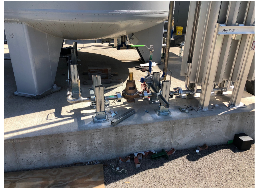
cryogenics piping installation on the outside LN2 dewar.
