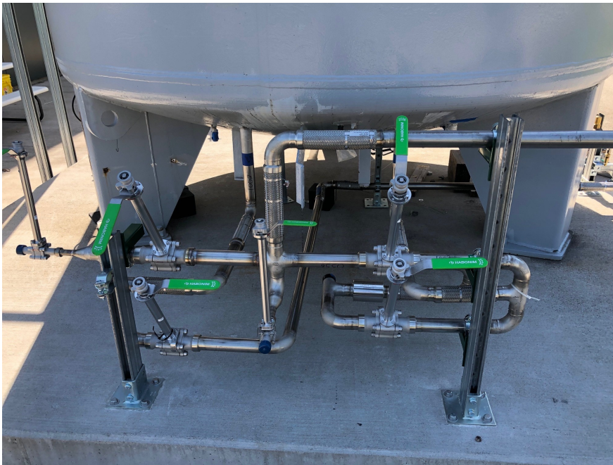
cryogenics piping installation on the outside LN2 dewar.
