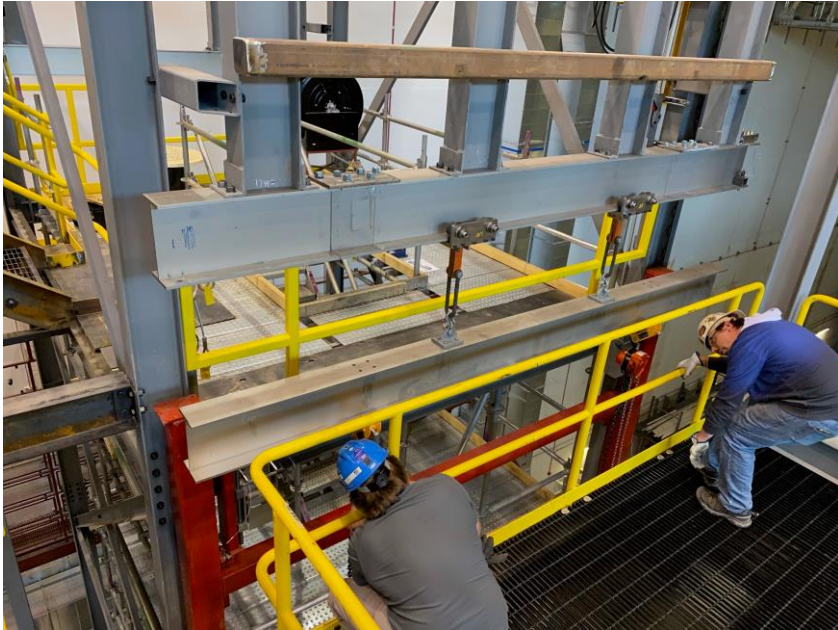
Taking the lower APA off the APA Tower
