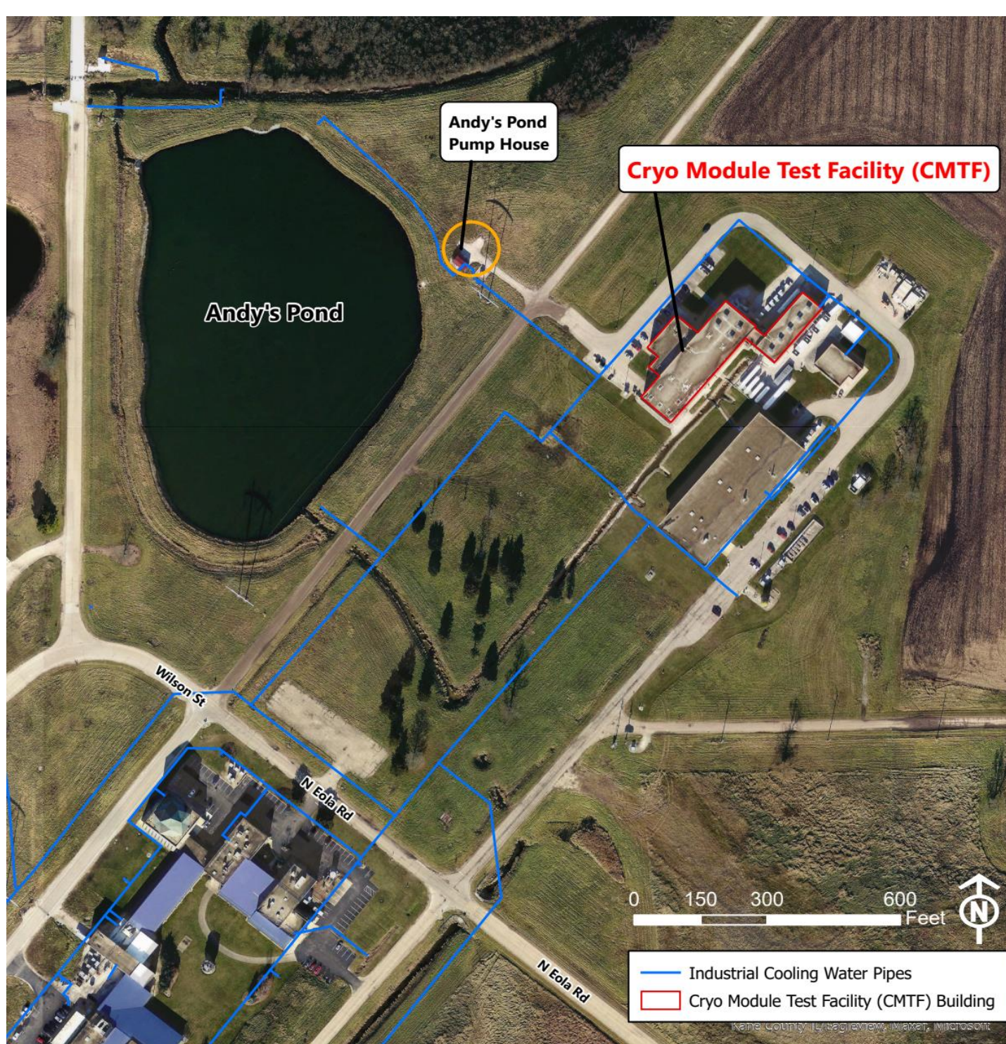
An overview of Andy's Pond, which supplies cooled water to the Cryo Module Test Facility (CMTF) building.
