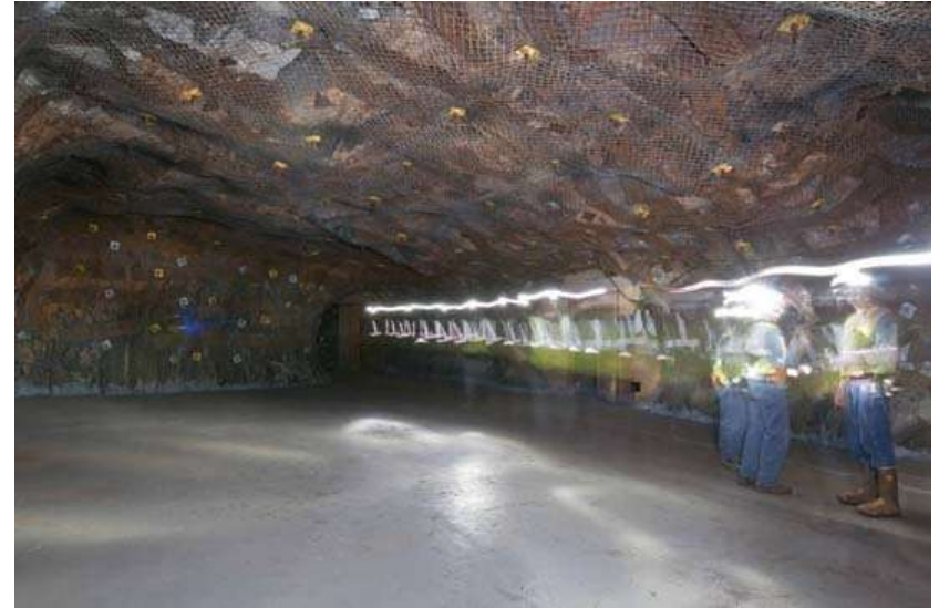
Davis cavern refurbished by South Dakota.
