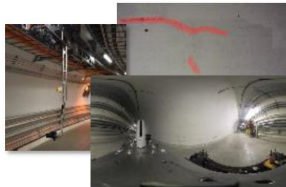
Tunnel structure monitoring
