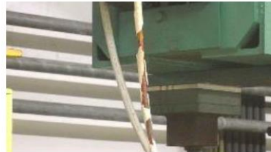
Cabling status inspection
