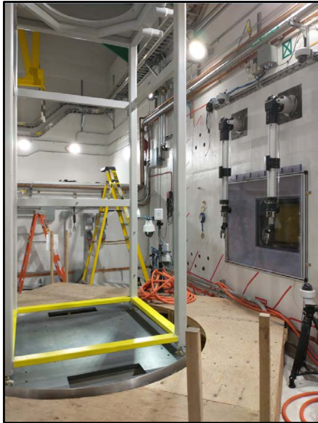
Equipment lift (left), manipulators (right)
