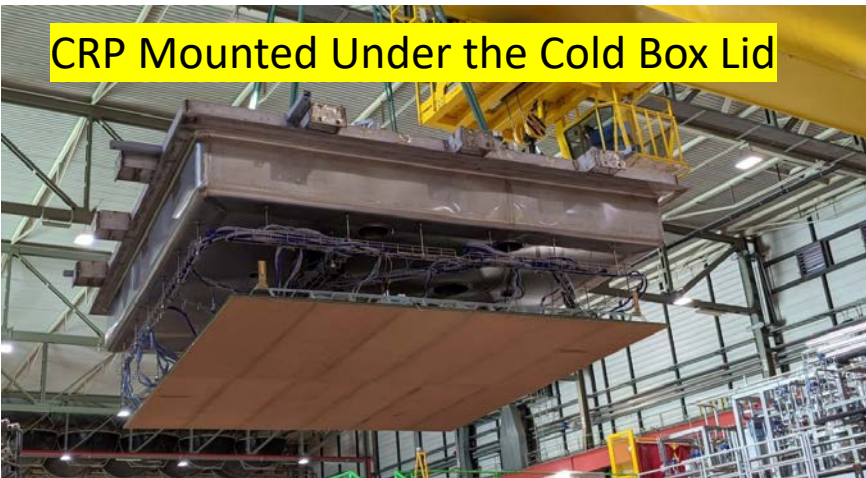
CRP Being Lowered into the Cold Box
