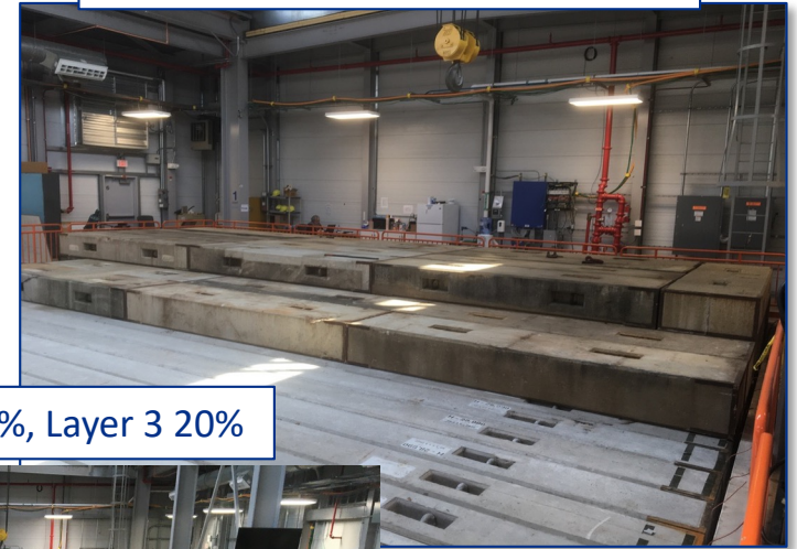
End of April: Layer 2 started
