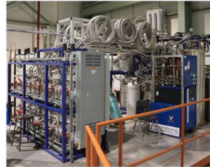
Quantum Technology Helium Recovery 200 L / day capacity – self sustaining
