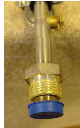
VCR connector of the cryomodule cooling circuit
