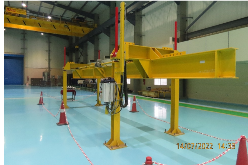
Jacking system installed at high bay
