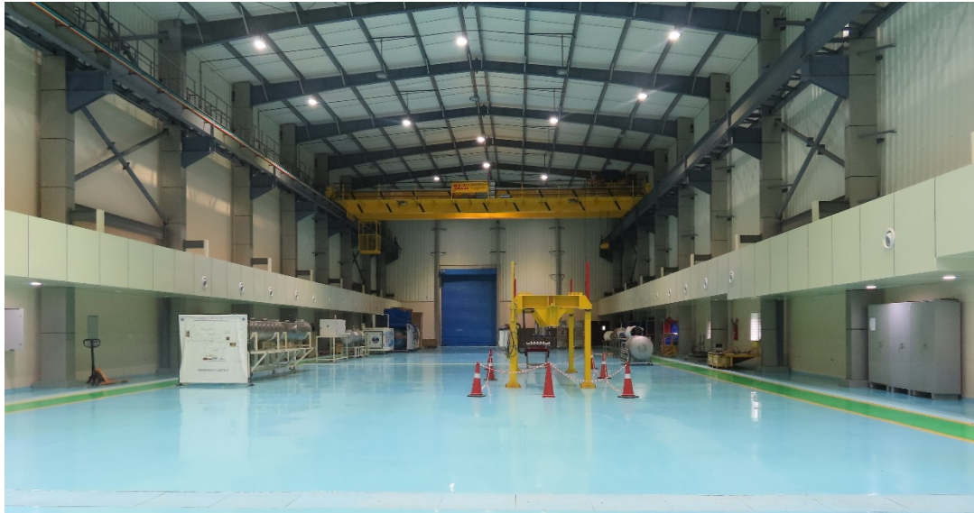
High Bay Area of CM Building 84m x20m
