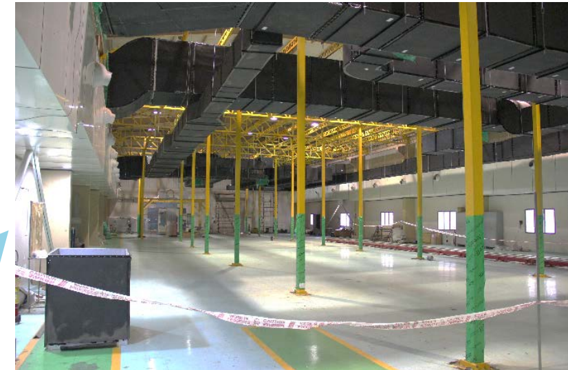
Cleanroom under construction
