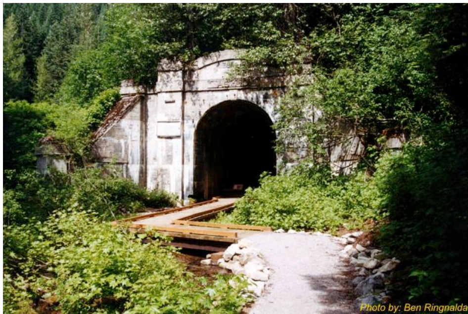
FIG. 2: West portal of the Old Cascade Tunnel.
