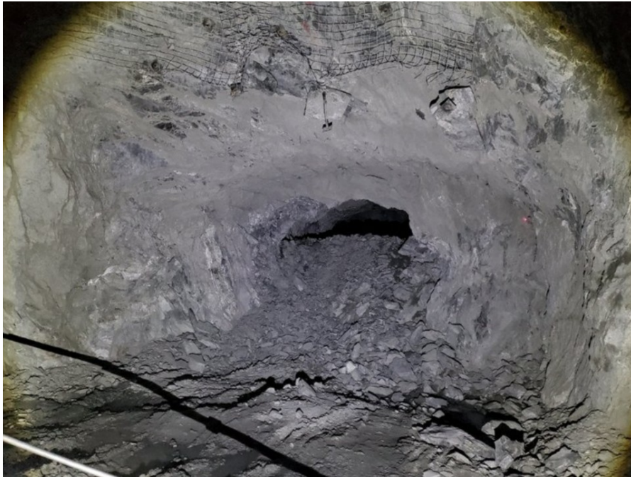
North cavern breakthrough January 2022
