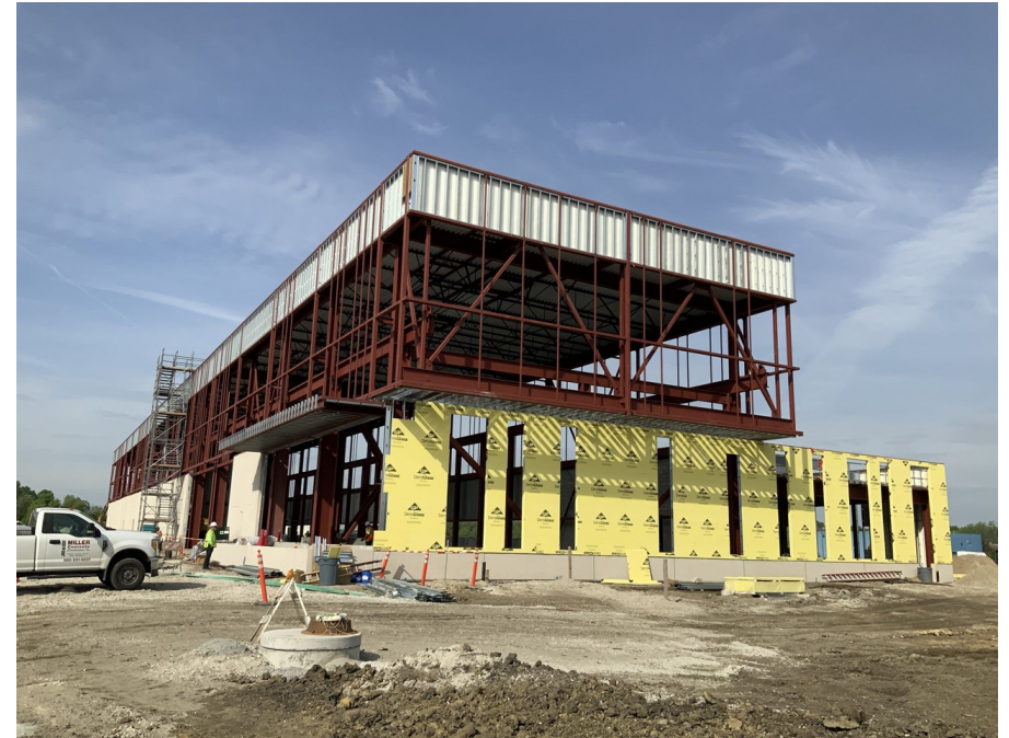
PIP-II construction May 2022
