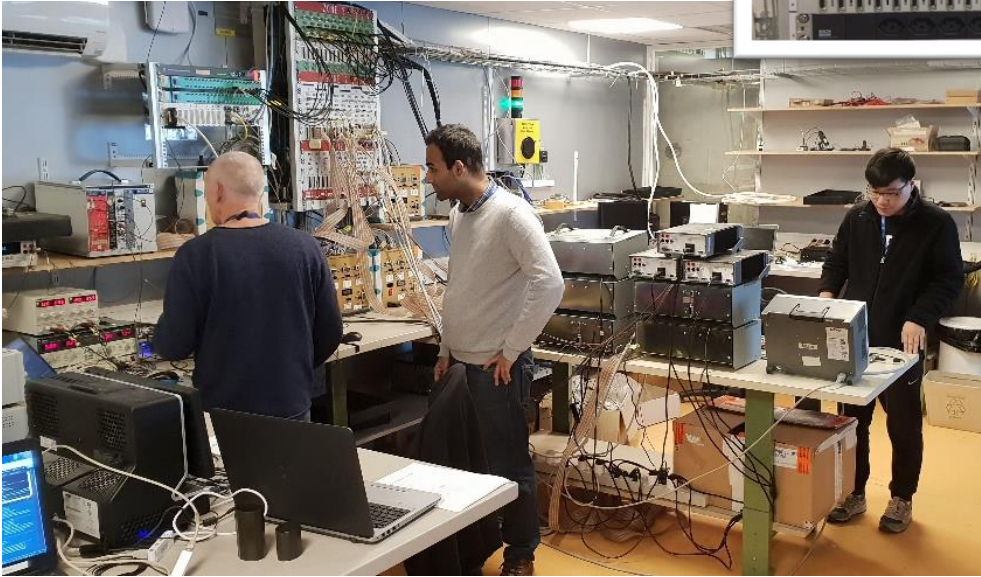
IRRAD Control Room
