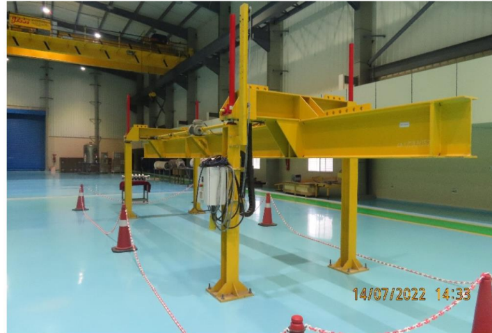
Jacking system installed at high bay
