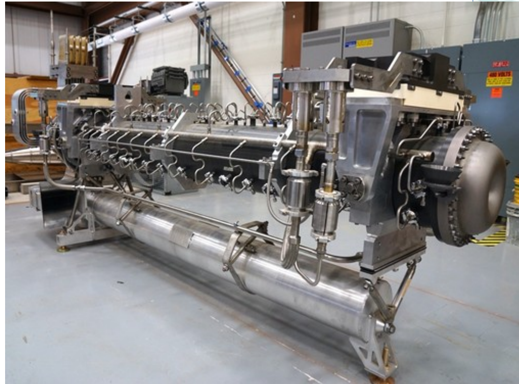
MW-capable horn (installing during 2020 shutdown)
