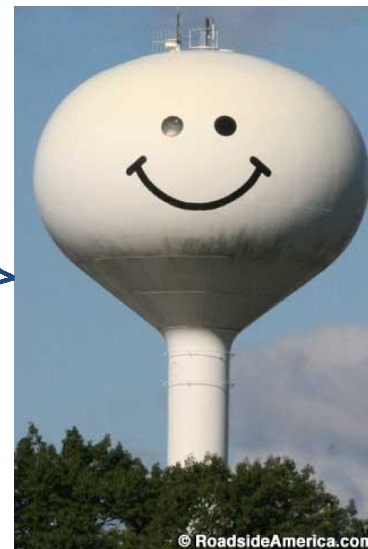
Figure 2: Example Water Tower
