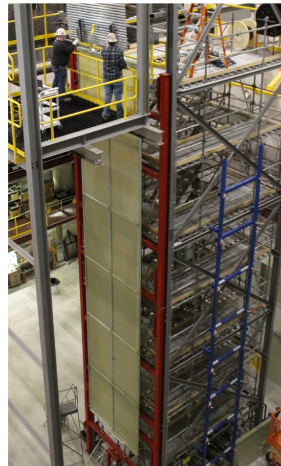
Fall 2020: 12m tall FD1 full height CPA installation
